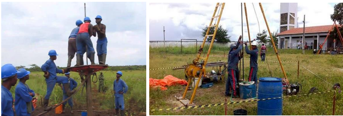
Figure 9 Banka drill rig and the diesel-powered YBM-05 drill rig respectively
